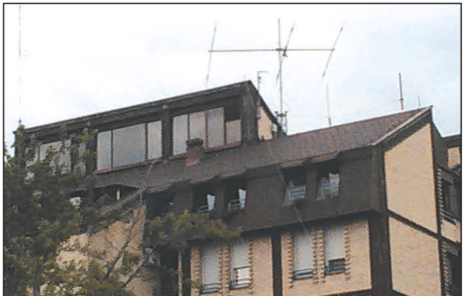
These rooftop antennas were key to YT8A's fine score.
