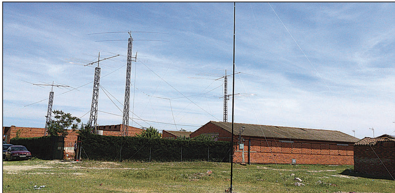
The impressive antenna farm at ED1R.
